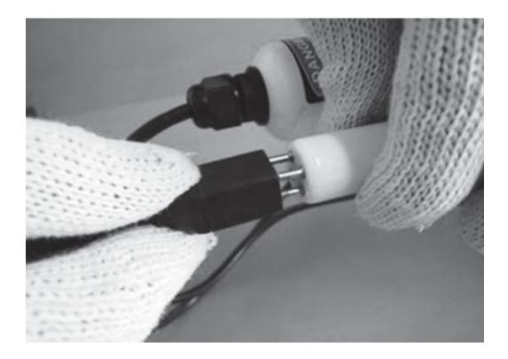
6. Withdraw lamp from quartz sleeve carefully. Be sure to withdraw lamp straight out without angling until completely clear of quartz sleeve.
