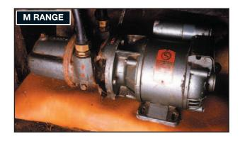
Installed over 40 years ago at a Welsh Farm, this MS pump from the M range is transferring water from a 15 feet deep well, along 20 yards of 1" diameter pipework to a 100 gallon tank. Activated by a float switch in the store tank, the pump typically stops and starts 3 times an hour.
